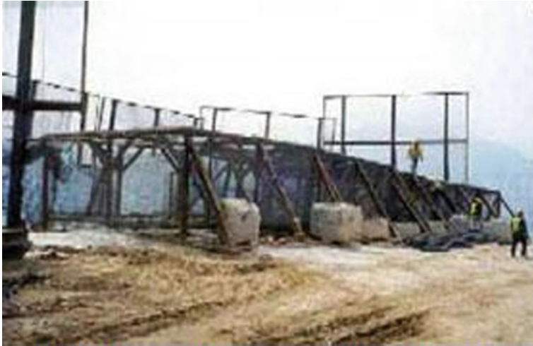
Fig. 11.10 Blasting cages with counterweight
