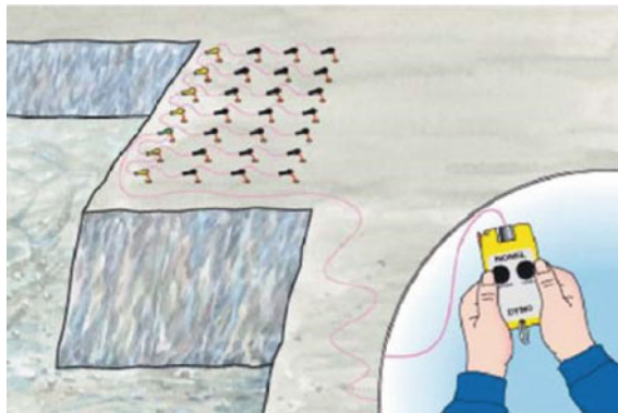
Fig. 4.21 Firing a blasting round using a blasting machine (Dyno Nobel)
