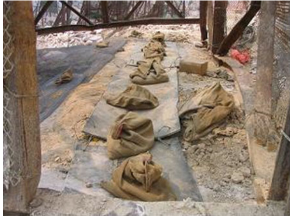
Fig. 11.32 Covering on the presplitting holes
