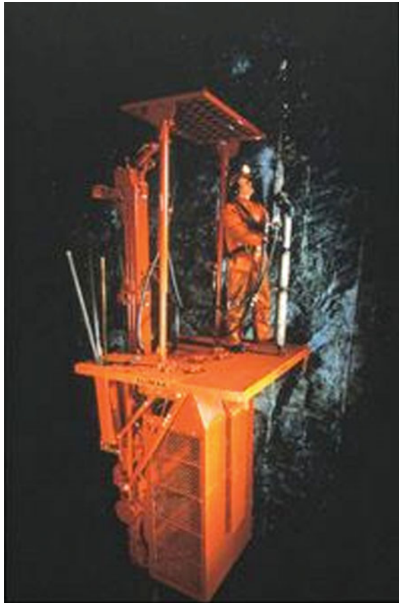
Fig. 16.13 Drilling on Alimak platform (reproduced by permission of Atlas Copco.)
