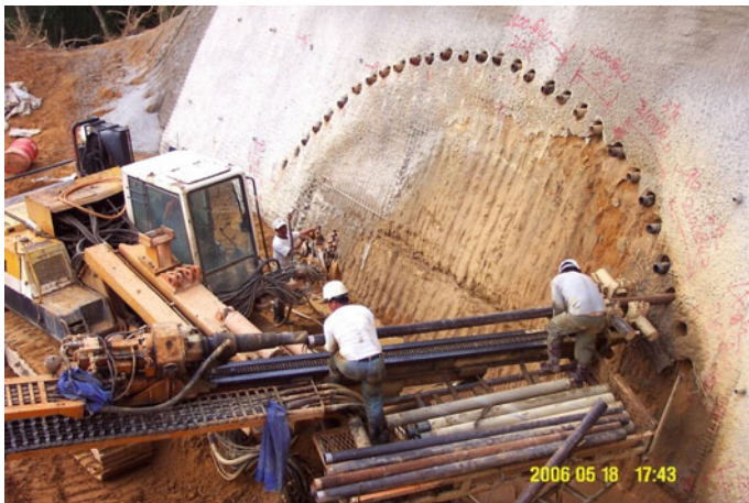
Fig. 21.38 Pipe screening for tunnel portal excavation Source http://mitac.sptc.com.tw/
