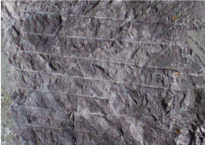
Fig. 17.1. Tunnel rock face formed by smooth blasting
