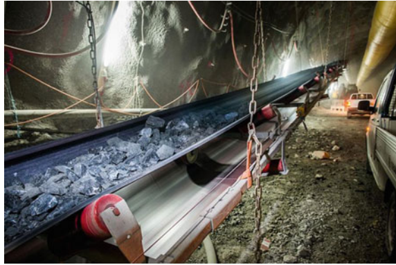
Fig. 19.10 Conveyor belt was used in Norway 14.3-km-long Solbakk tunnel (Reproduced from Ref. [5] by permission of TunnelTalk)
