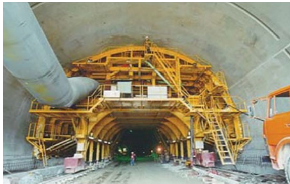
Fig. 21.50 Steel arch self-propelled traveling lining form for in situ concrete lining
