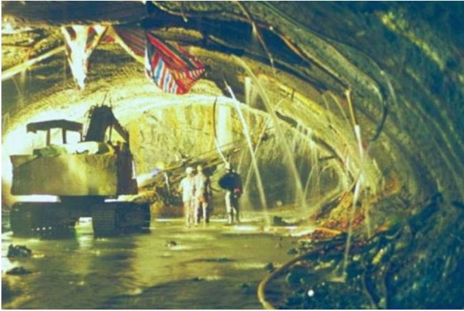
Fig. 1.44 Groundwater affects tunnel construction
