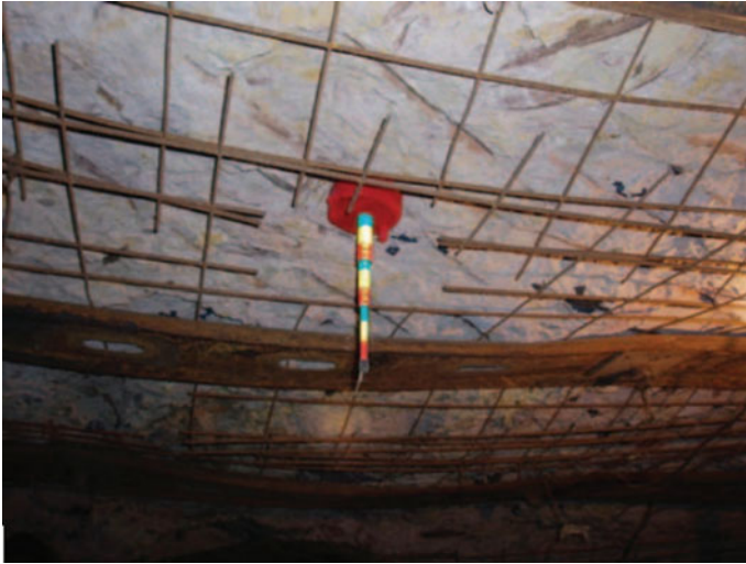
Fig. 22.4 Typical installation of triple height telltale
