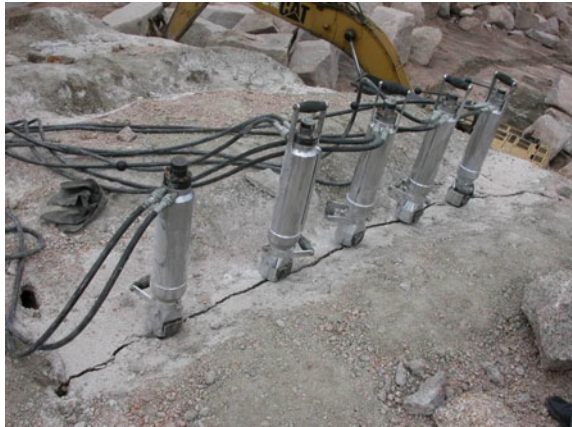
Fig. 7.6 Multi-gun hydraulic rock splitter is working (Courtesy of China Flying Technology Ltd.)
