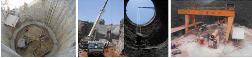
Fig. 19.15 Simple equipment for shallow shaft sinking operation
