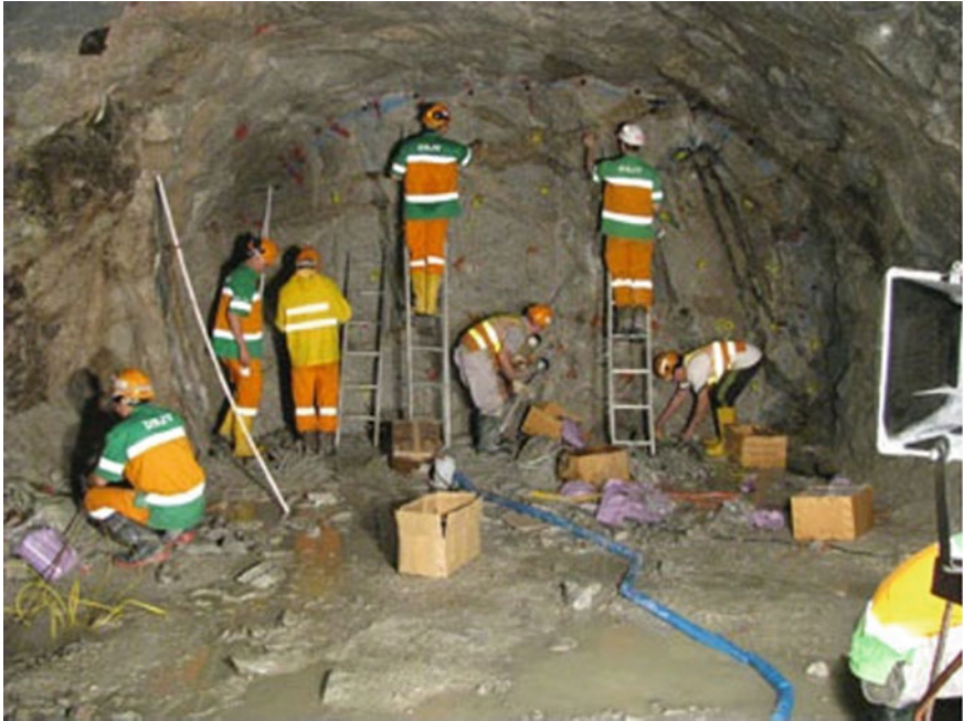
Fig. 16.16 Manual explosive charging in face. Source www.dsd.gov.hk/others/HKWDT/
