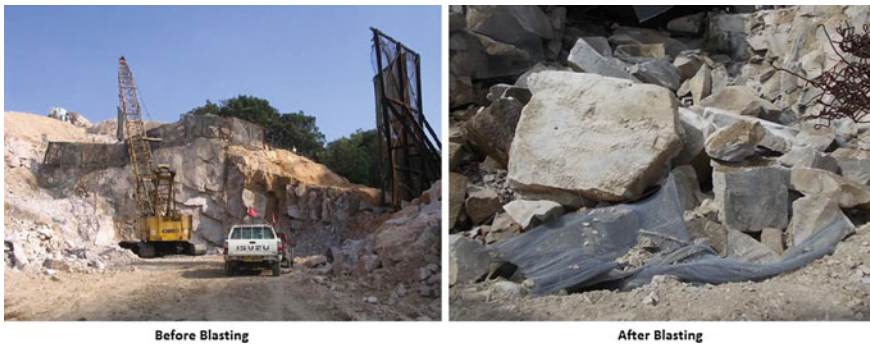
Fig. 1.35 Bad fragmentation by blasting hard and less jointed rock mass
