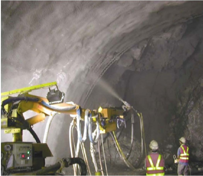
Fig. 21.33 Shotcrete manipulator works in tunnel
