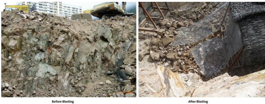
Fig. 1.36 Good fragmentation by blasting weathered and highly jointed rock
