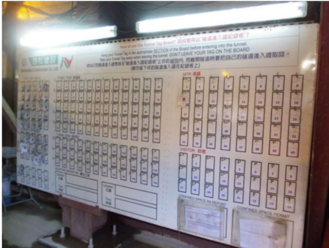
Fig. 23.1 Board of tally system which is located at the entrance of underground construction for check-in and checkout of all personnel
