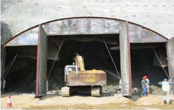
Fig. 23.8 Blasting door for tunnel blasting
