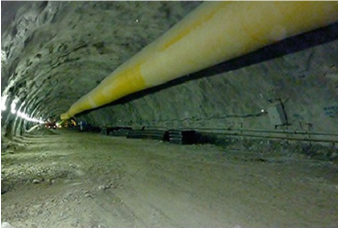
Fig. 20.3 Flexible smooth ducts made of plastic fabric for tunnel ventilation. Source www.hpcproducts.com
