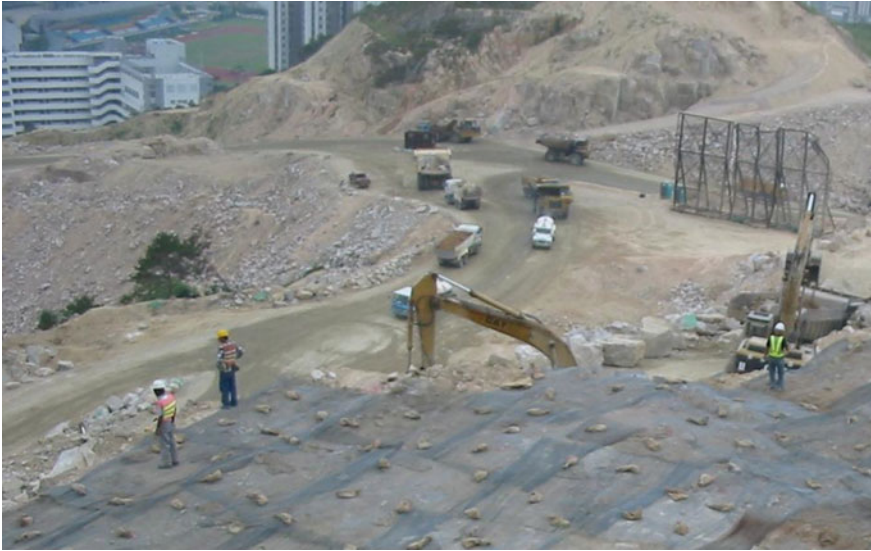
Fig. 11.8 Ground cover with wire mesh mats
