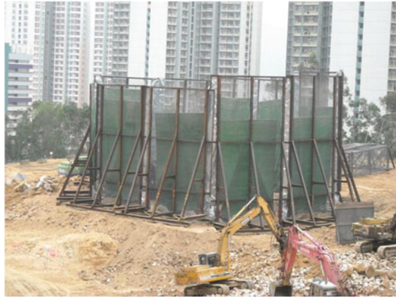
Fig. 11.34 Vertical screens covered with canvas as sound barriers are surround the blasting area
