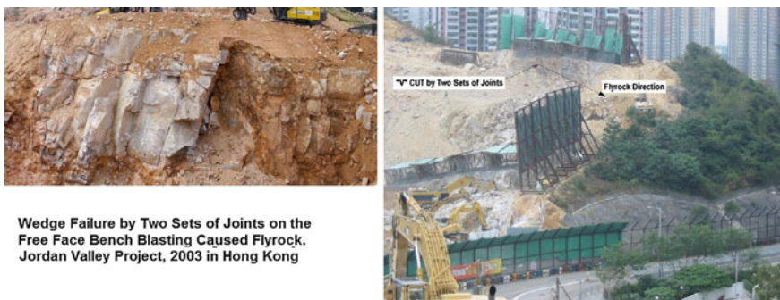
Fig. 1.38 Wedge failure by two sets of joints on the free face caused flyrock in blasting
