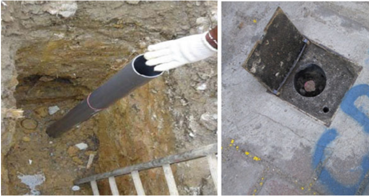
Fig. 22.9 Settlement mark for utility monitoring
