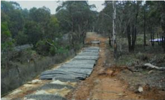
Fig. 9.5 Trench blasting with ground cover of rubber tyre mats
