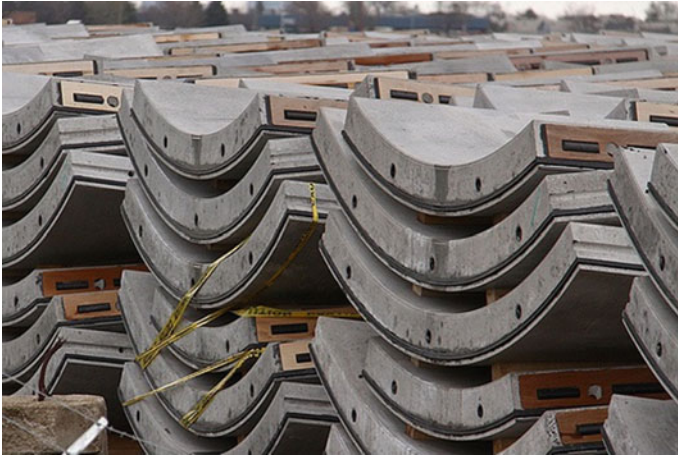
Fig. 21.45 Precast concrete segment for tunnel support
