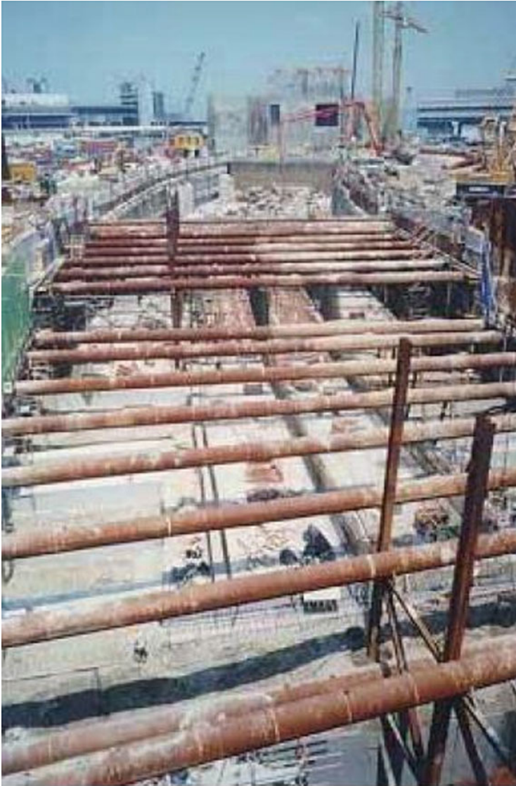
Cut and Cover Tunnel for the Airport Railway at the Central Reclamation in Hong Kong in Late 1996. Section of the tunnel pit formed by diaphragm wall and strutted by the use of steel tubes. The construction of the tunnel sections using in-situ method can be seen inside the pit.
