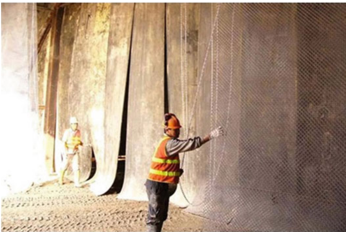
Fig. 23.9 Hanging waste rubber belt and wire mesh between the blasting door and the blasting face to reduce the impact to the steel door
