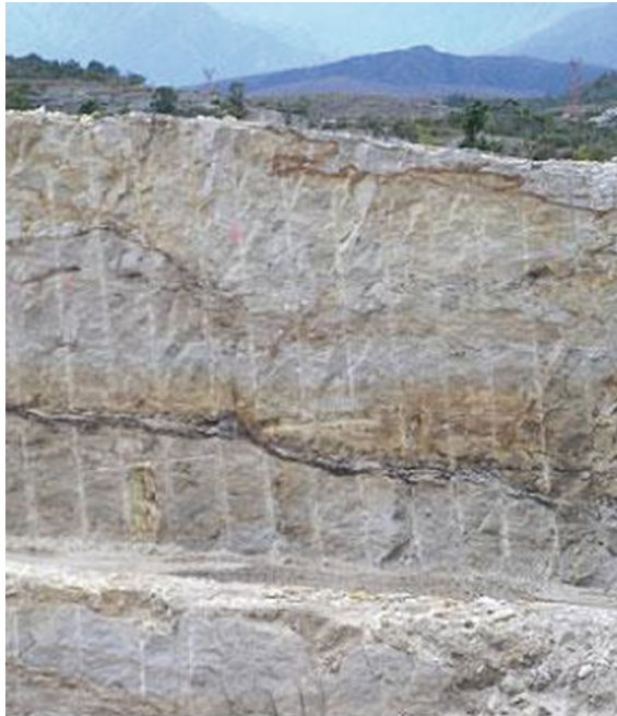
Fig. 10.4 Slope face formed by presplitting
