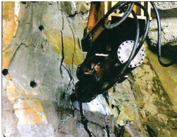
Fig. 14.2 Breaking tunnel rock with wedge hydraulic splitter
