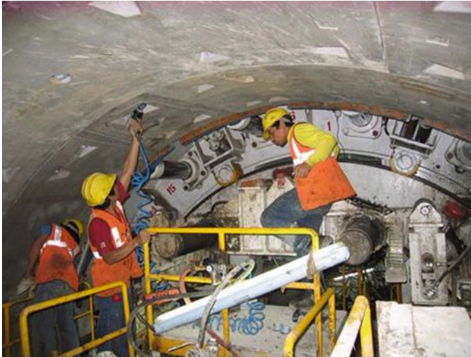
Fig. 14.29 Installation of segment lining for TBM tunnel
