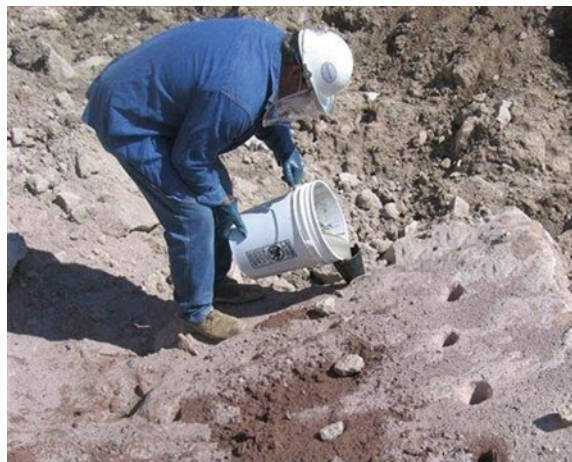
Fig. 7.11 Pouring cracking mortar to drillholes
